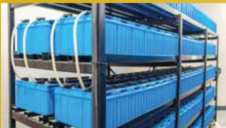
Example of standby batteries
